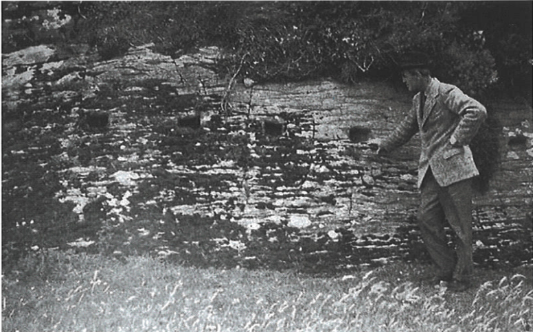
Plate III. Fish palace at Baltimore, Co. Cork, showing natural rock with holes for supporting press beams. (Source: Went 1945) Reproduced by permission of the Cork Historical and Archaeological Society ©.
