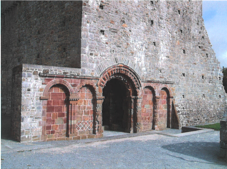
Plate II. Romanesque door with blind arcading on east wall at Ardfert Cathedral. (Photo: Isabel Bennett)
